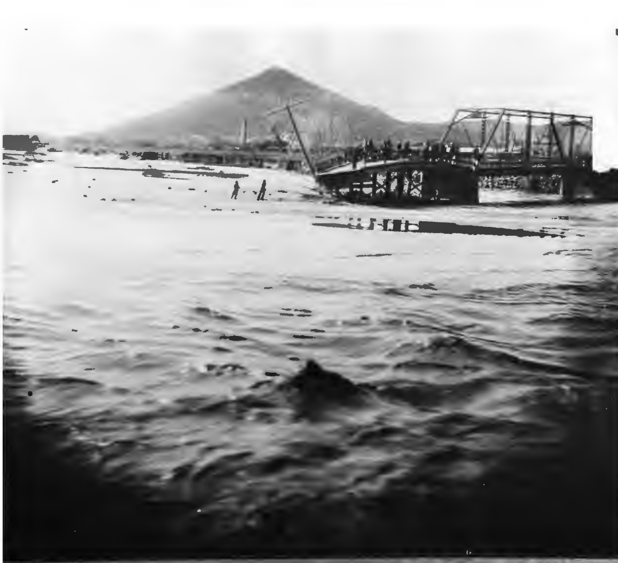
The Congress Street bridge over the Santa Cruz River near Sentinel Peak in Tucson washed out during flooding in 1915.
