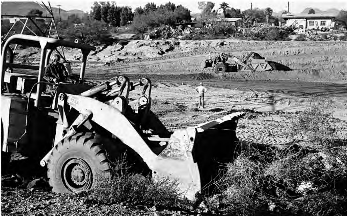
After years of waiting, crews began clearing debris and channeling the Santa Cruz River in November, 1977, and constructing what would become a 14-mile river park.
